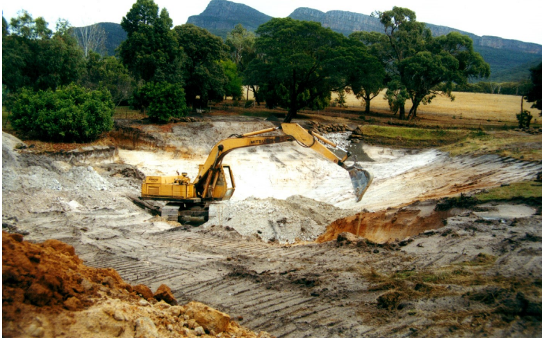
Excavating the Valley Dam and building the bank
