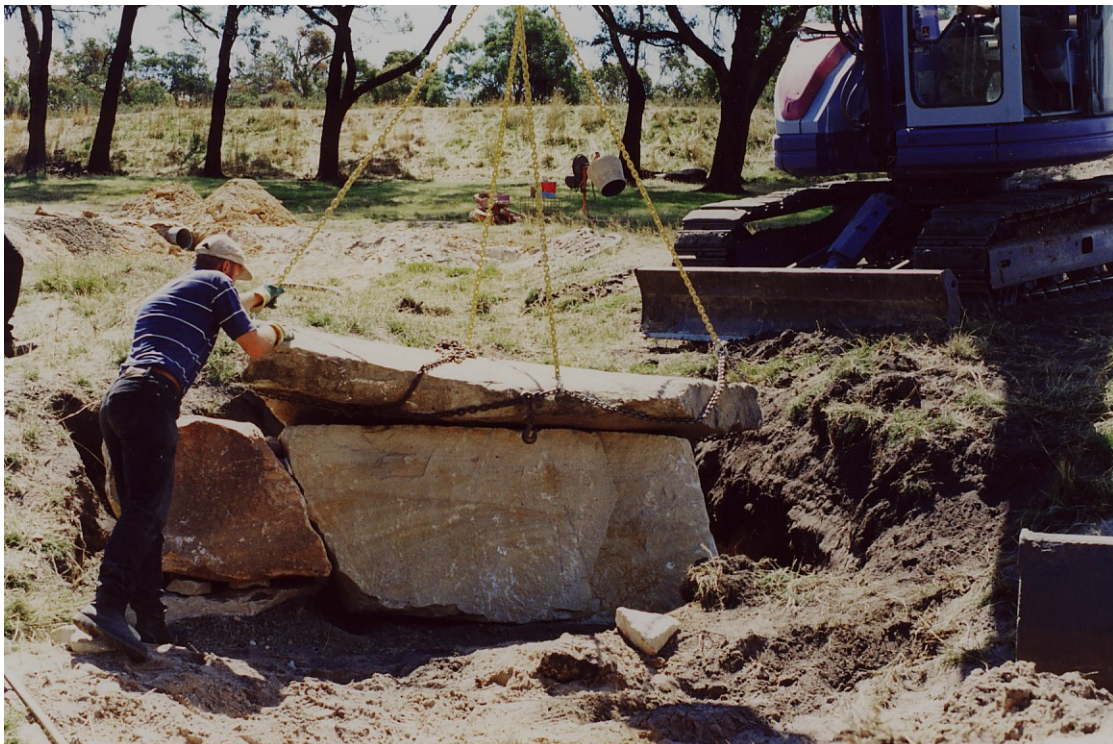
Laying the top stone slab of the waterfall, part of the Cascades
