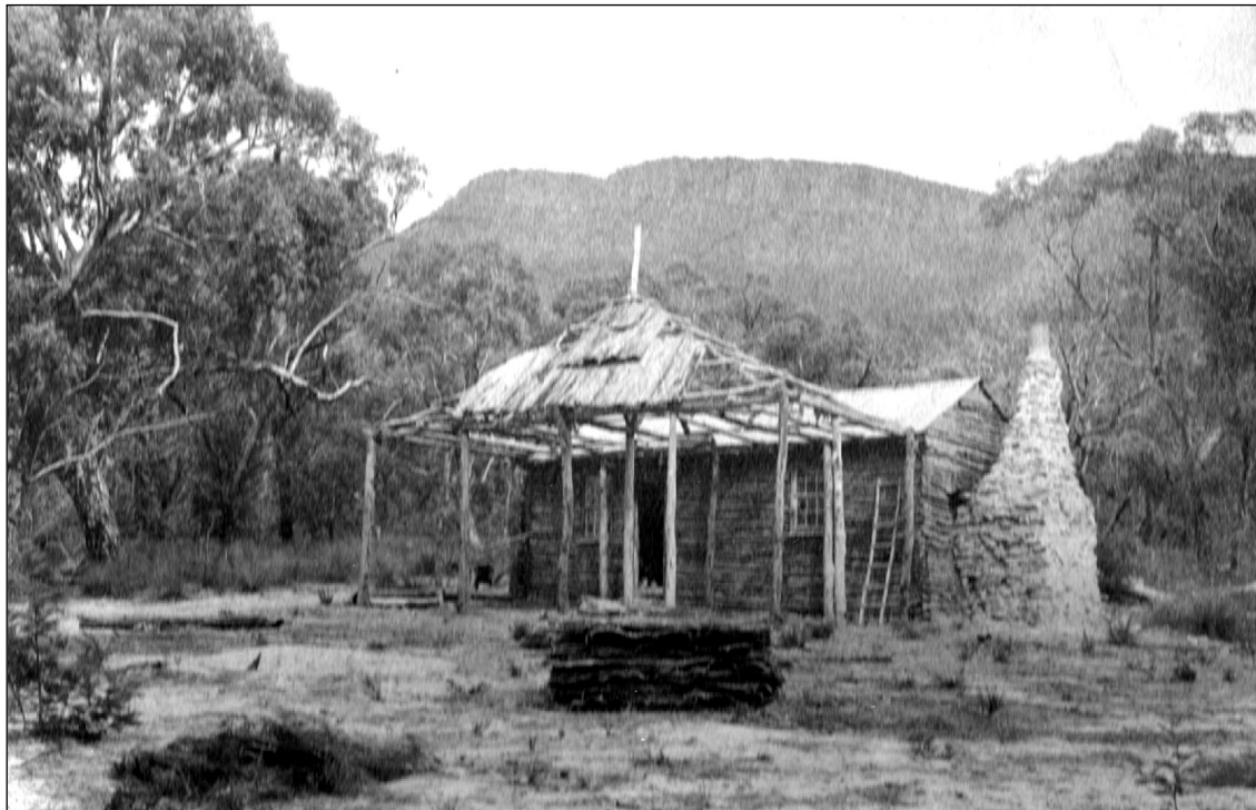
"The Ranch" at "The Mount". — It had wattle and daub walls, and iron roof. The structure in front made of bush timber has a bark roof.
