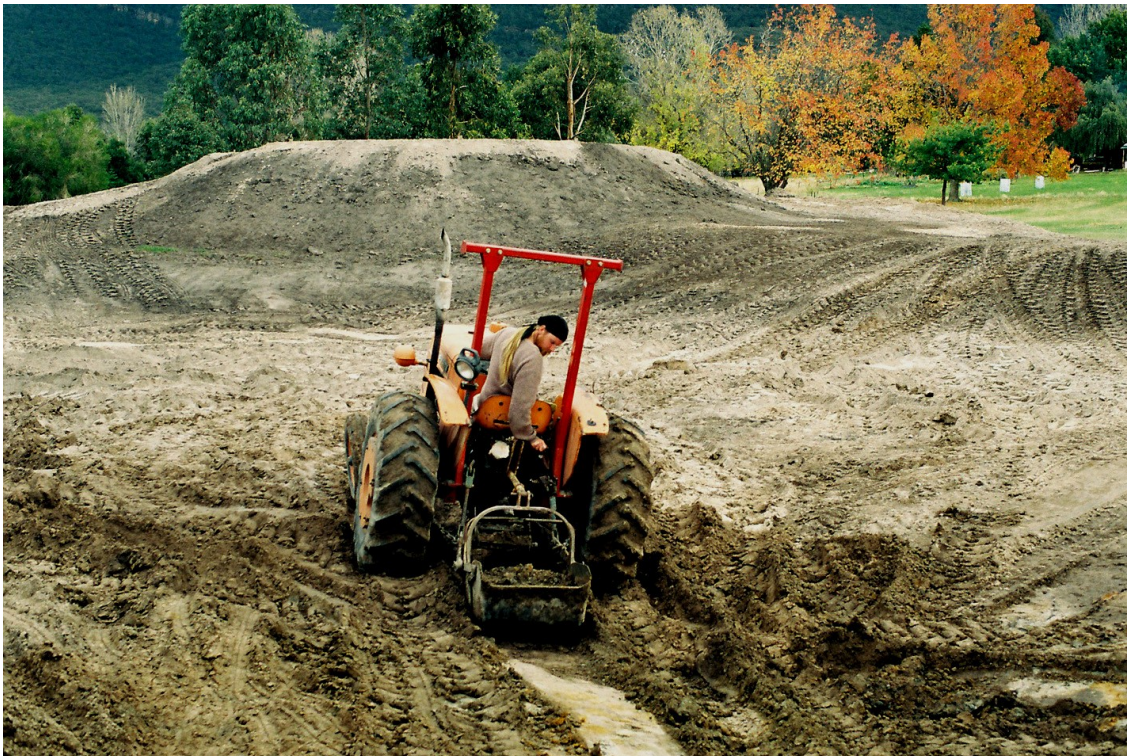
Building the Observatory Dam with the Fiat tractor and Ferguson back scoop
