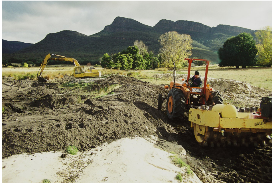
Building the wall of the Fourth Dam; Aidan on the fiat tractor compacting the bank, 2002
