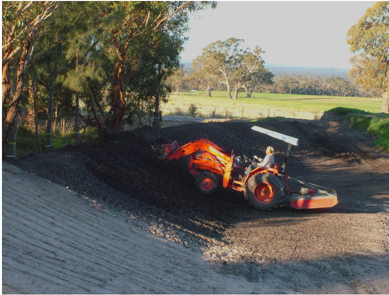
Finishing the north wall of Blue Lake South with good compacting soil
