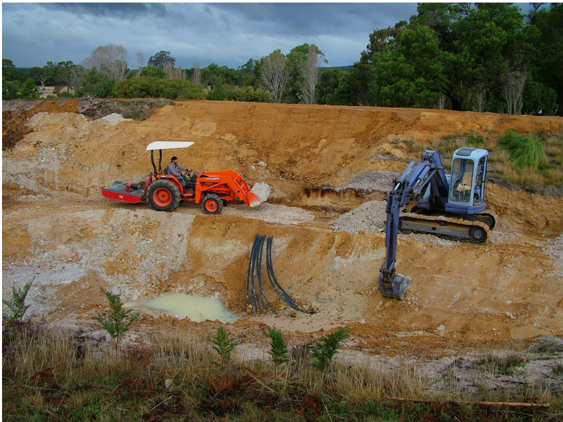
Lining the south bank of the Fire Wetlands with clay
