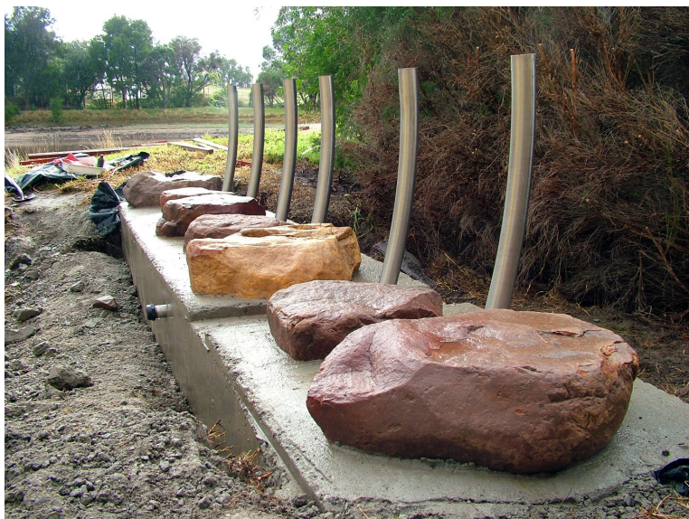
Above: The completed overflow with stepping stones. Below: Removing sand and building up the north wall with soil.
