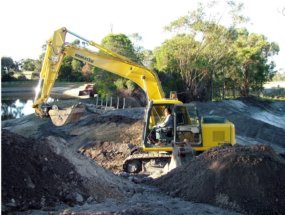
Aidan using excavator to form passage between Blue Lake and Blue Lake South, 2008
