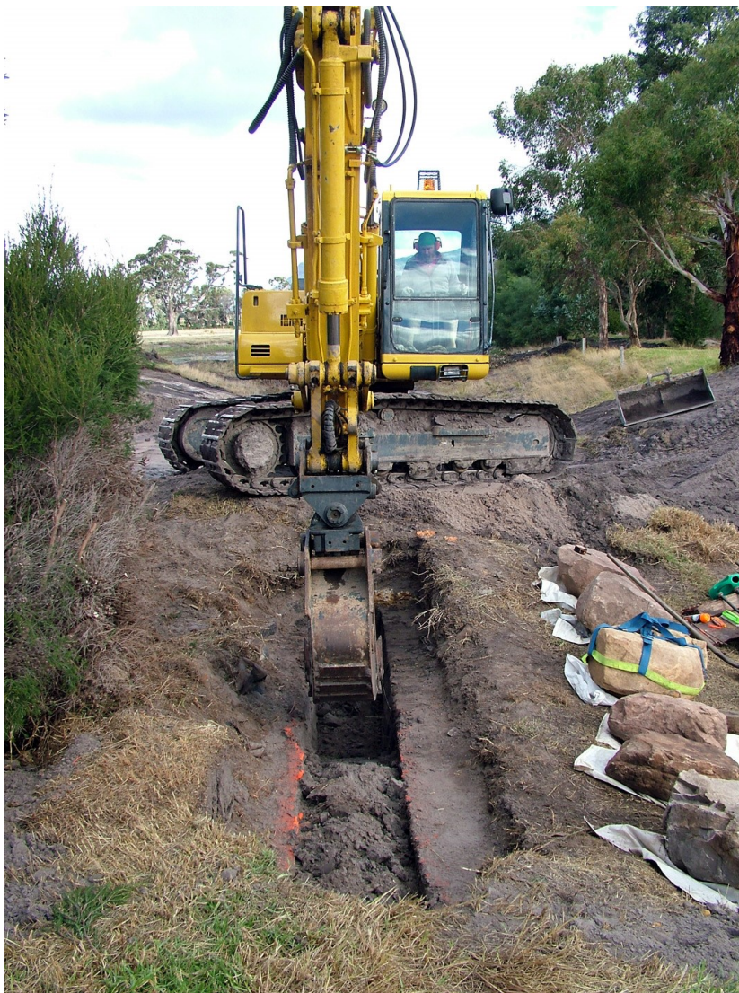
Aidan using the excavator to dig the concrete foundation for the overflow
