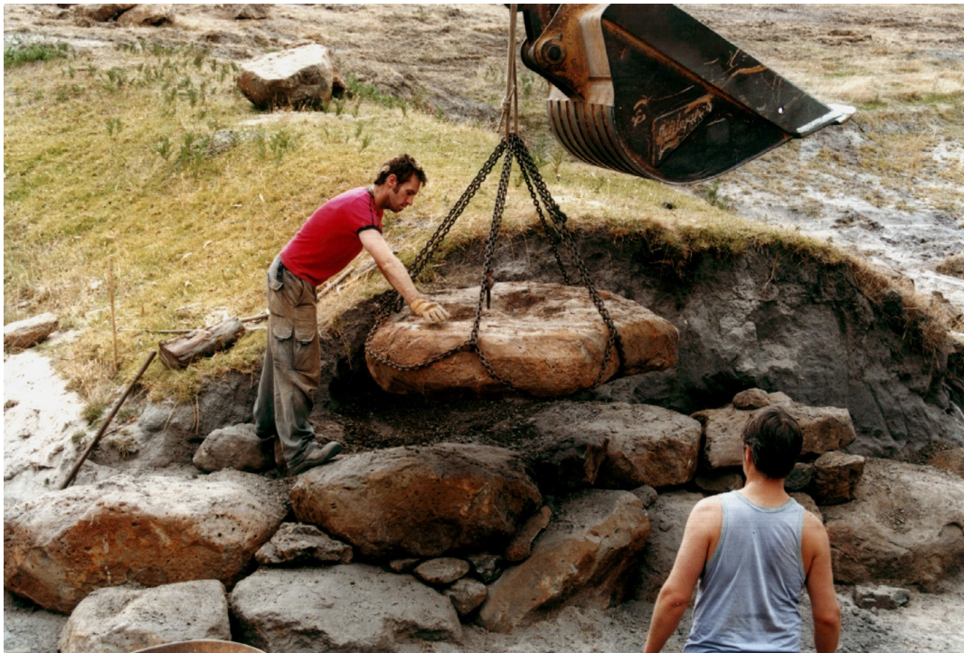
Building the dry stone wall on the bank at the west end of Valley Dam
