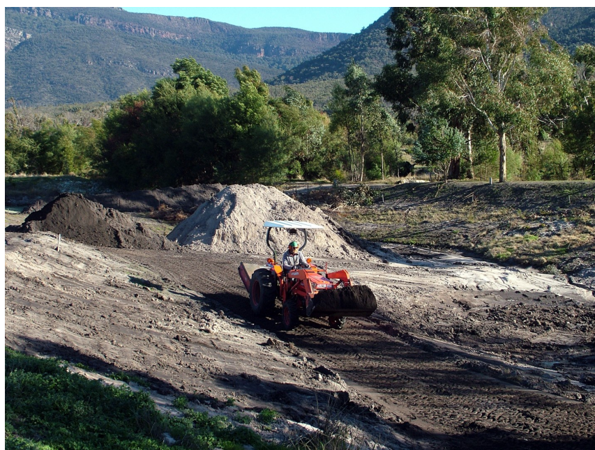
Above: The completed overflow with stepping stones. Below: Removing sand and building up the north wall with soil.
